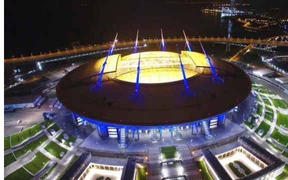
Figure 1. Gazprom Arena in Saint Petersburg
