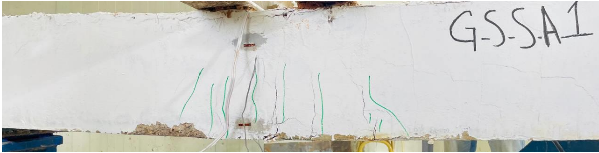
Figure 3. Beam GSSA1 after failure.
