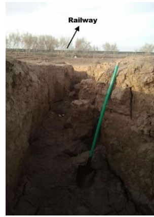
Fig. 4. Sampling location and the position of the created channels in relation to the railway
